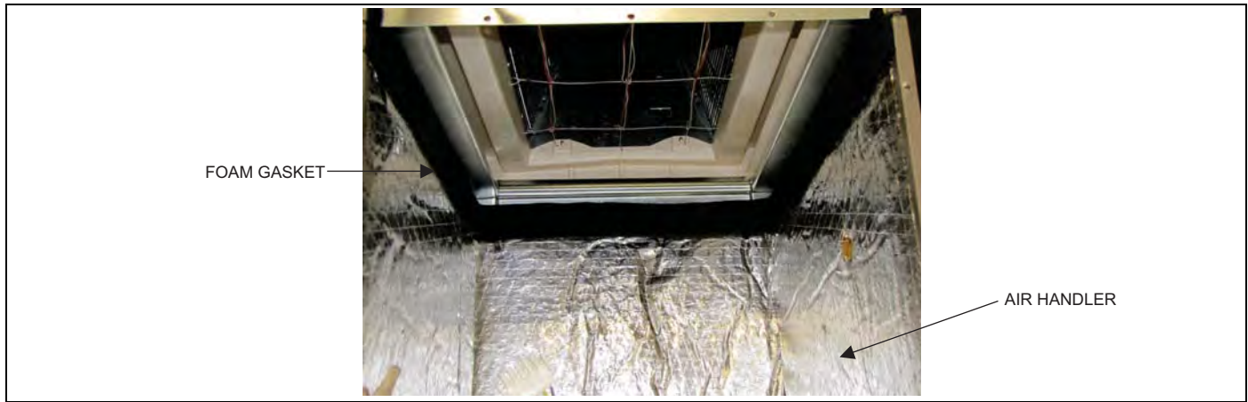
FIGURE 4: Gasket Location
