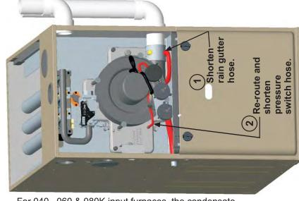
drain is plumbed toward the right casing outlet from the factory.
