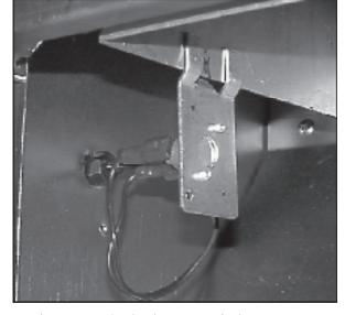
Figure 1: Flame Rollout Switch
