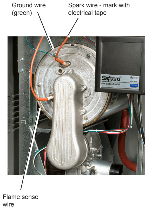
Fig. C5-6 - Disconnect the wires on the front plate of the heat exchanger
