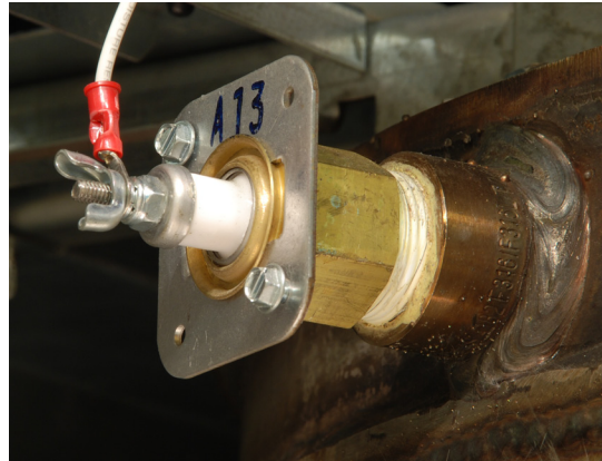
Fig. B6-1 - Removing the probe for the low water cutoff
