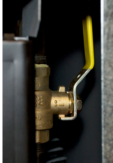
Fig. C5-2 - Gas shutoff valve (typical)
