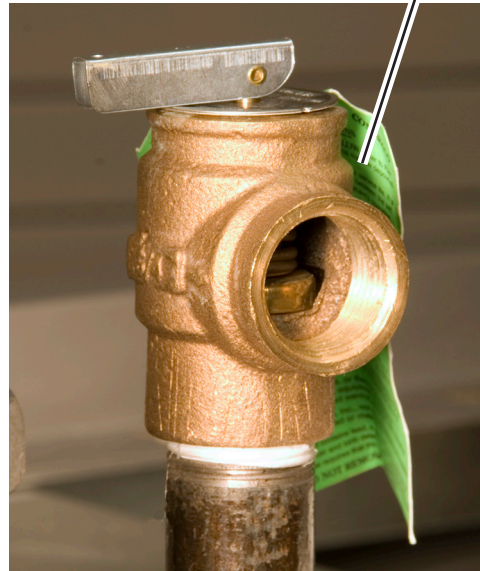
Fig. B35-1 - Pressure relief valve (typical)
