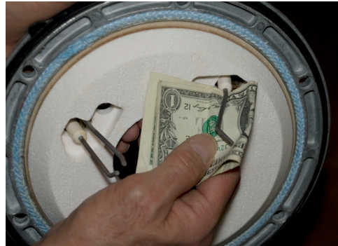
Fig. B37-1 - Correct way to clean the flame sensor
