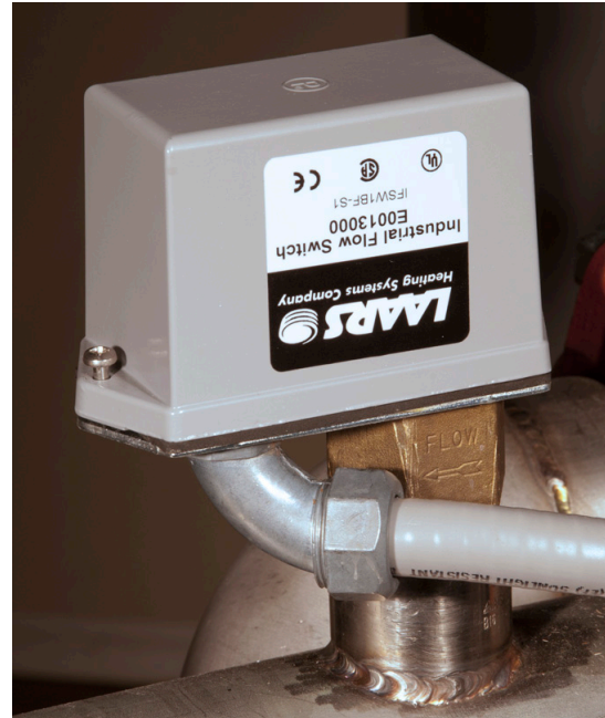
Fig. B9-1 – Typical flow switch installation
