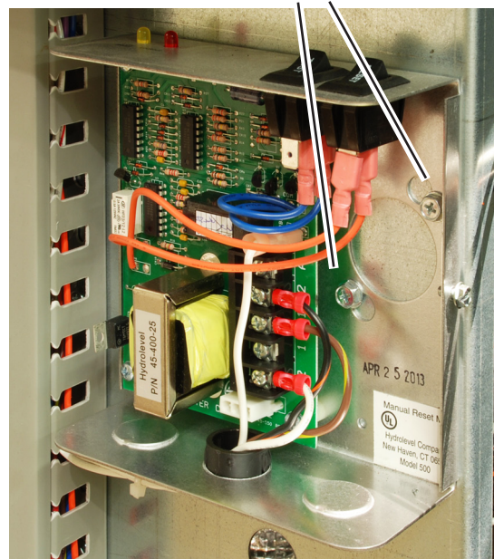
Fig. B6-3 - Control for low water cutoff with cover removed
