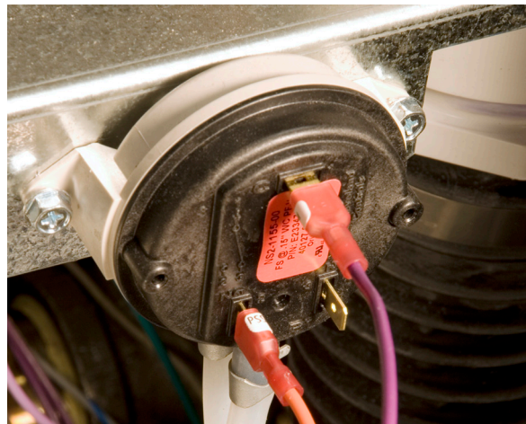
Fig. B21-1 - Air pressure switch (typical)
