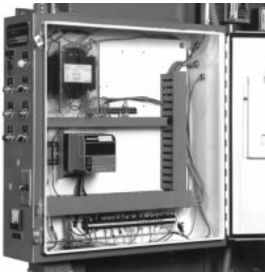
Fig. 8—Electrical panel installation.
