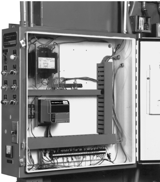
Fig. 8. Electrical panel installation.
