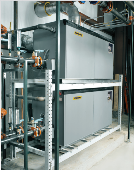
Space saving, rack mounted Pennant boilers with Laars Linc intuitive control system.
