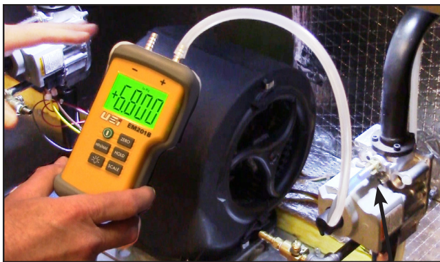
Figure 36. Measure Supply Gas Pressure
