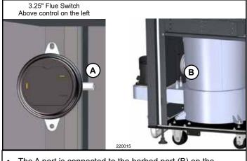
The A port is connected to the barbed port (B) on the condensate dish.
